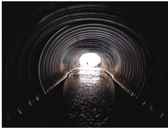
Video Image on Project 1, Harpster, showing significant change in pipe deflection near outlet.
