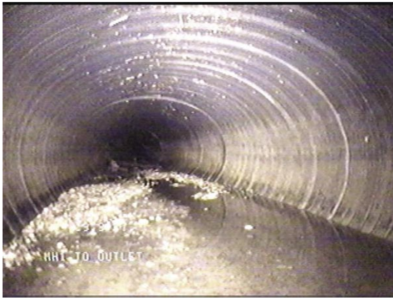
Video Image on Project 2, US 68/KY 80, showing approximately 20% deflection.
