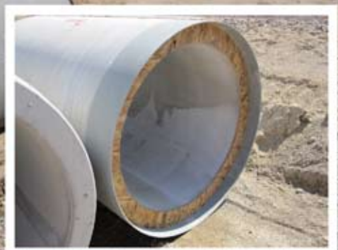
72" Class V Jacking Pipe, Lehi, UT Photo: Mountain States Concrete Pipe Association
