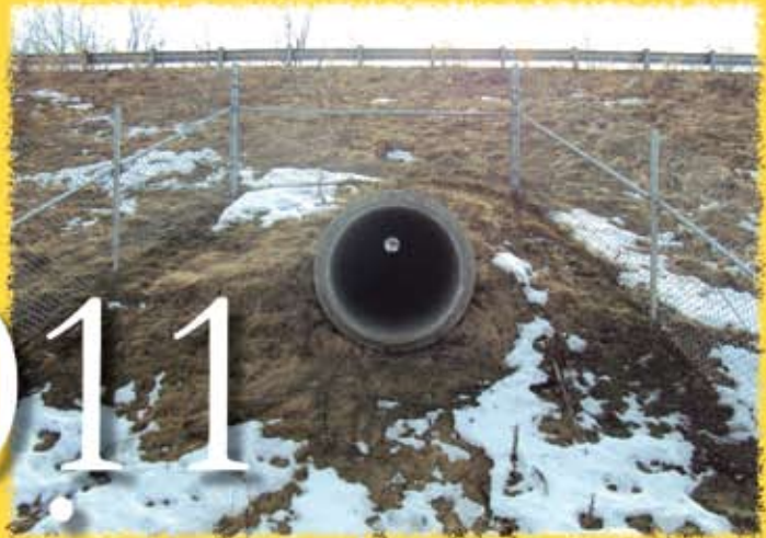
42" Wildlife Crossing, North Kingtown, RI Photo: Rhode Island DOT
