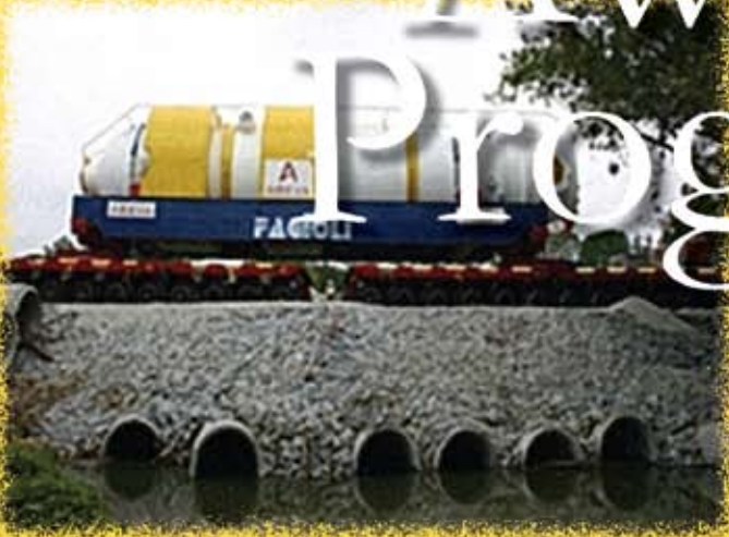
48" Class IV RCP Bridge Bypass for 510 Ton Steam Generator Photo: Oldcastle Precast, NE Pipe Group
