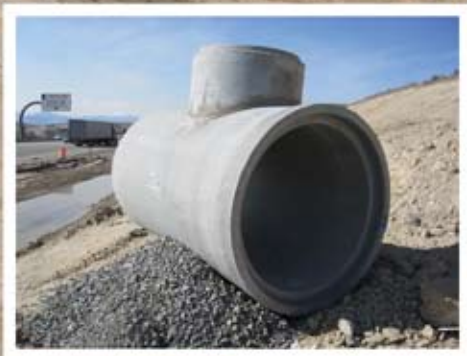
SR-92 Drainage Manhole "T", Lehi, UT Photo: Mountain States Concrete Pipe Association
