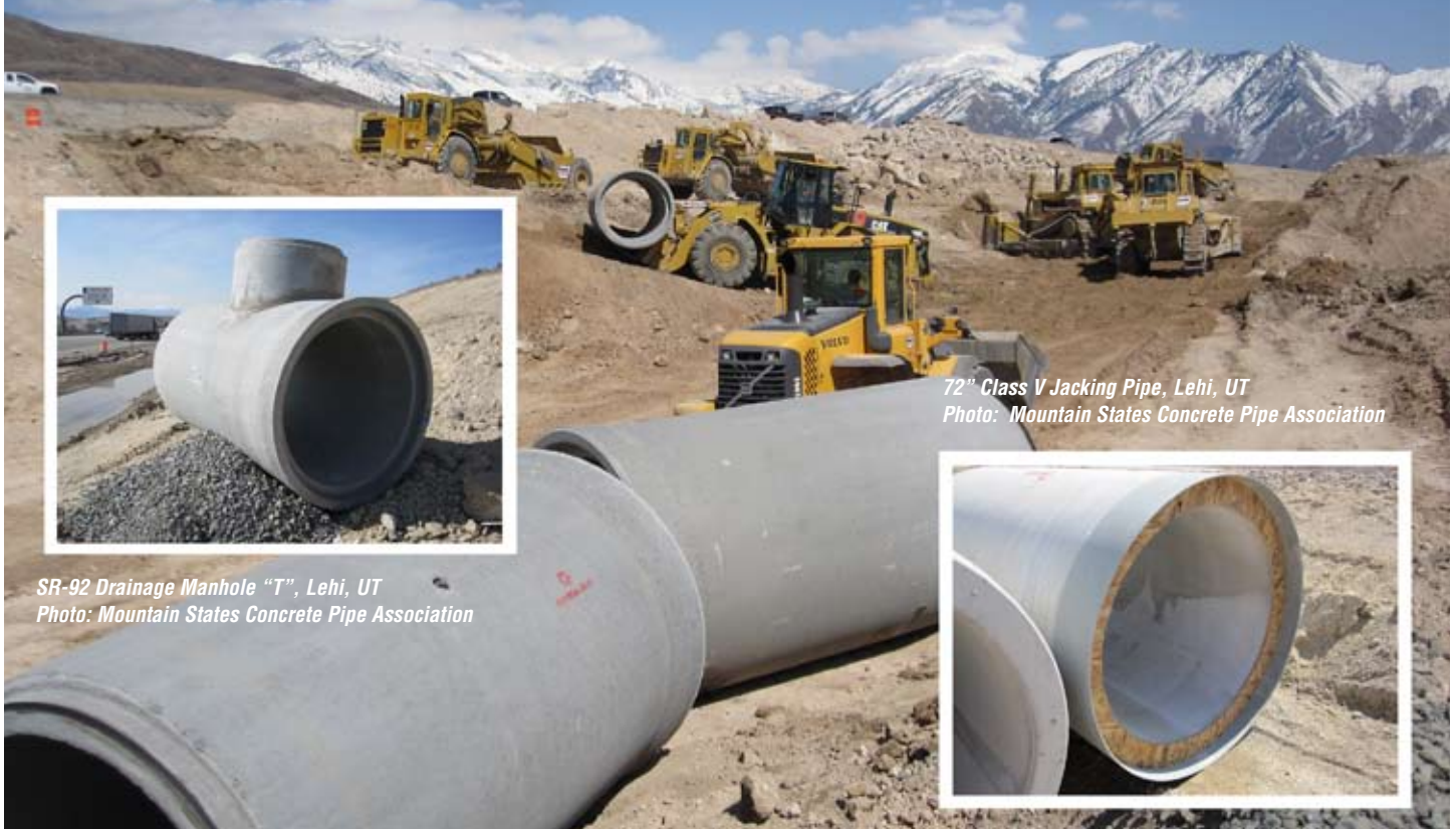
SR-92 Drainage Construction, Lehi, UT Photo: Mountain States Concrete Pipe Association
