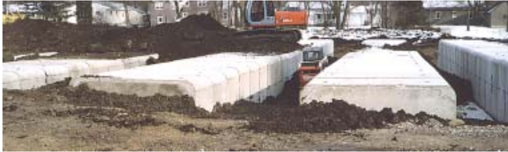
Five parallel lines of 12-foot x 8-foot precast concrete box sections used for stormwater detention under parking lot and lawn.
