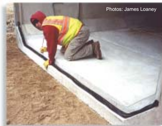
Joint mastic ensures water tightness.
