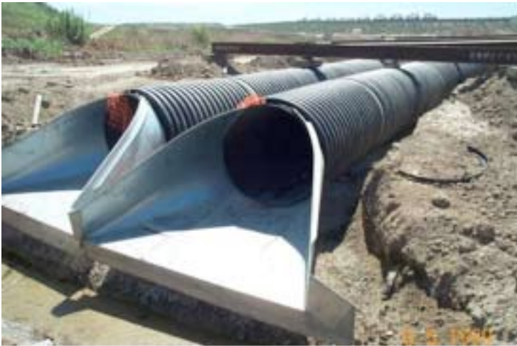
Figure 6. Otay River 60in HDPE
