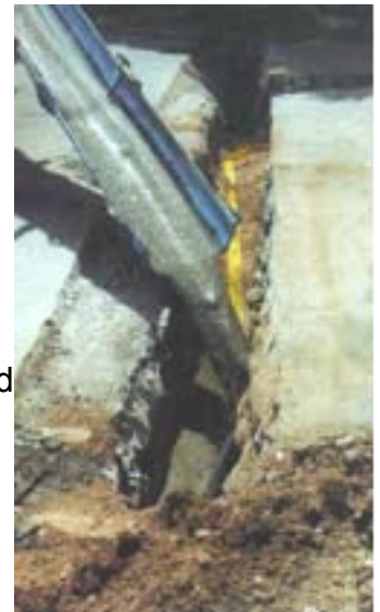
Figure 3. Flowable Fill Installation
