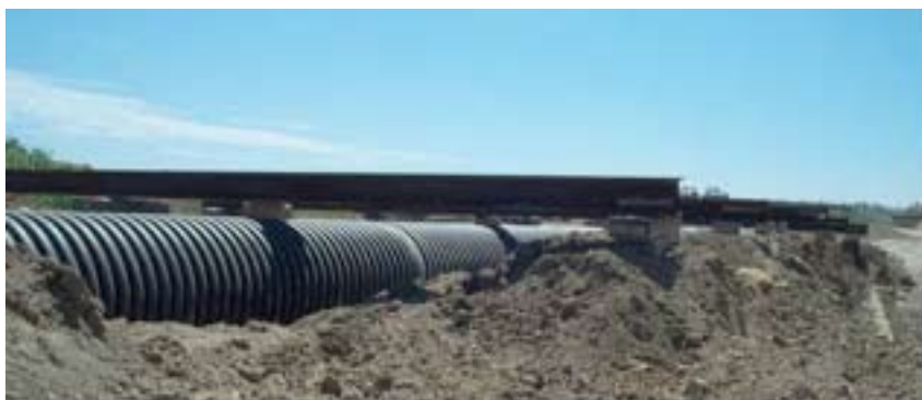
Figure 5. Large Steel Tie-Downs for HDPE Pipe
