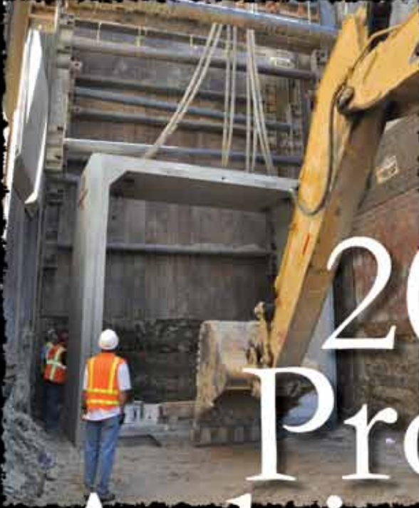
14' x 14' Precast Box Culvert, Sandy, UT Photo: Mountain States Concrete Pipe Association
