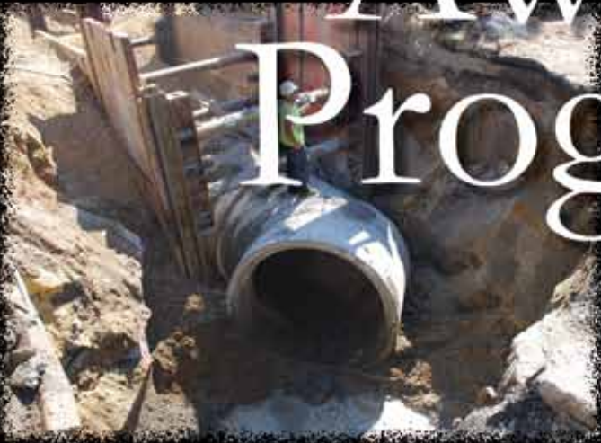
84" RCP Elbow, Philadelphia, PA Photo: Oldcastle Precast, NE Pipe Group
