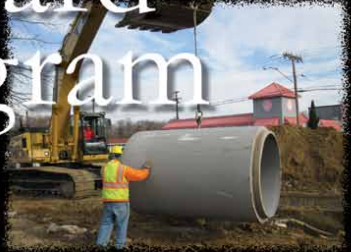
66" RCP, Somers Point, NJ Photo: Oldcastle Precast, NE Pipe Group
