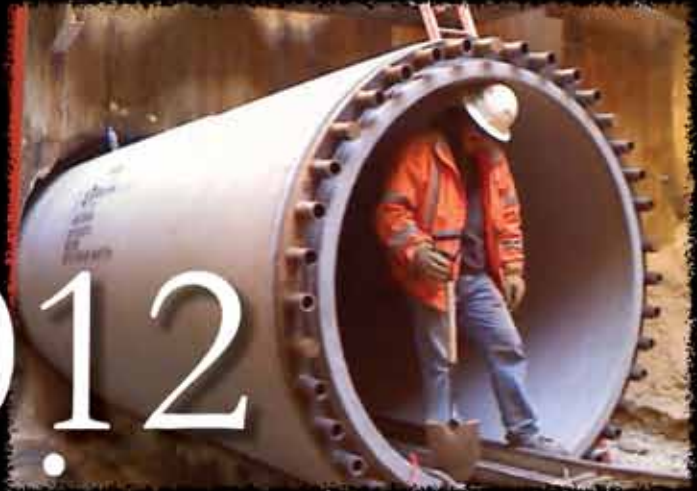
66" Jacking Pipe, Herriman, UT Photo: Oldcastle Precast
