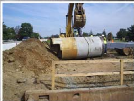
Jacking Shield Attached to 53 Inch RCP, Newark, DE Photo: Rinker Materials Concrete Pipe Division (CEMEX)
