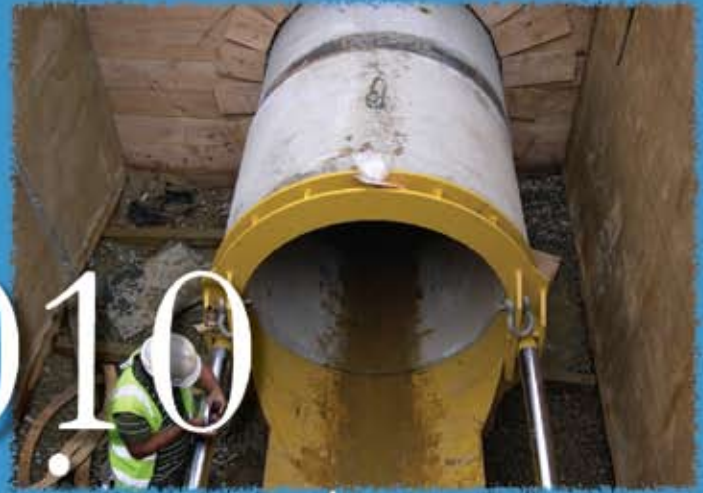
54 Inch Jacking Pipe, Newark, DE Photo: Rinker Materials Concrete Pipe Division (CEMEX)
