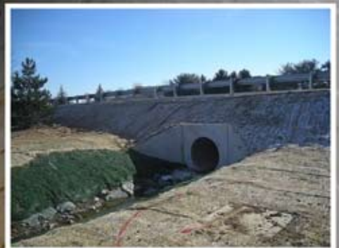
Outfall of 54 Inch Jacking Pipe, Newark, DE Photo: Rinker Materials Concrete Pipe Division (CEMEX)
