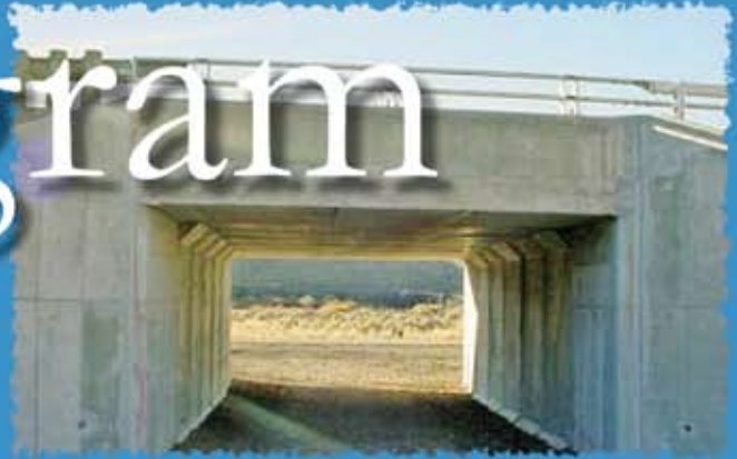
20 Foot x 12 Foot Box Culvert, Nugget Canyon, WY Photo: Wyoming DOT
